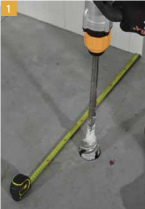
1 Measure and drill locations for anchor fixings.
