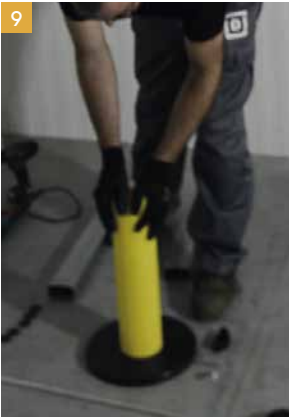
9 Assemble wall reinforcement arm components.
