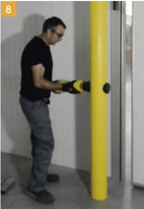
8 Fix reinforcement arm to vertical post.
