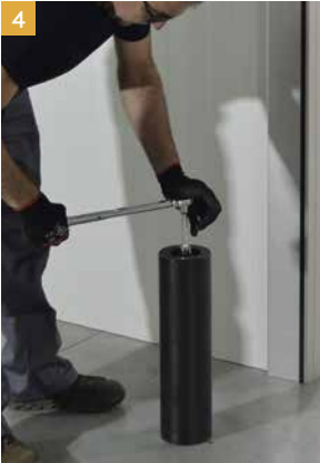
4 Locate anchor base and fix securely.
