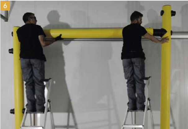
6 Position and fix horizontal beam to posts.
